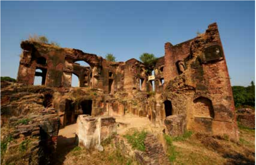
Aam Khas Bagh Sirhind
